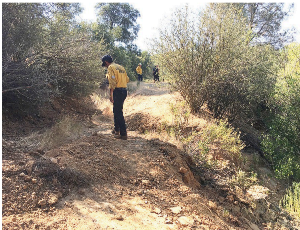
Restoration crews were quickly on the scene at Stockton Creek Preserve following the French Fire.
