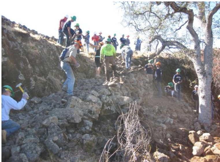
Building a rock access ramp for a Table Mountain trail
